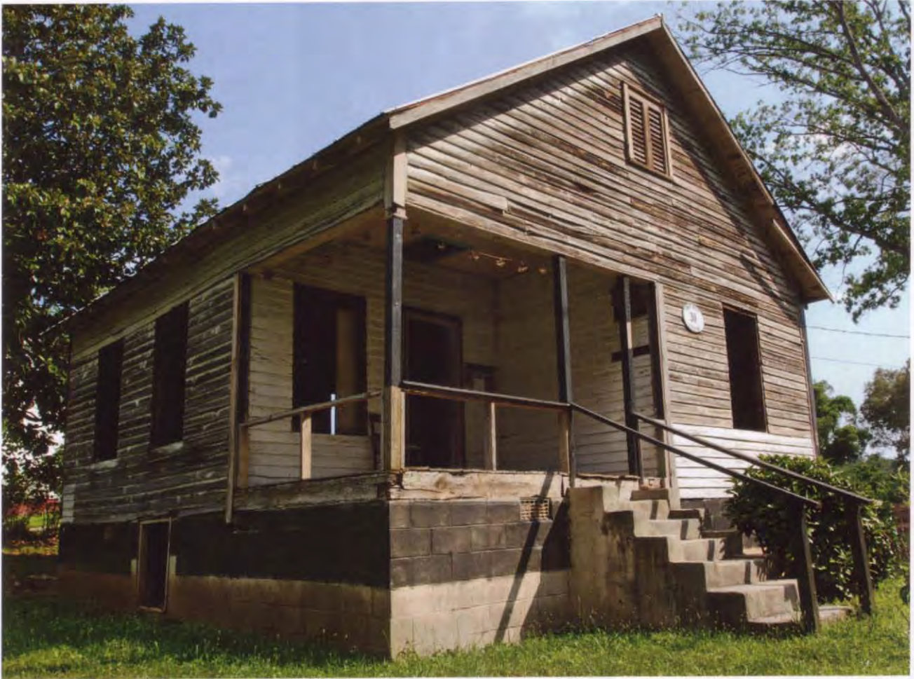
The McIntyres plan to replicate the home's original clapboard with lumber from a local mill. They will then paint the house to match its 1930s appearance.
